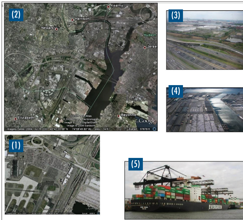
Figure 2-17: Exit 14, Newark, NJ.
