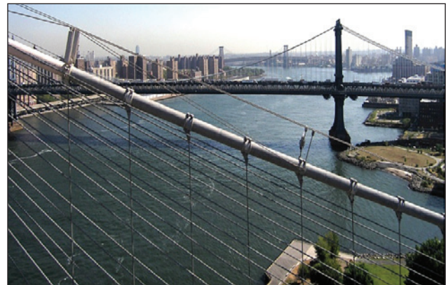
Figure 3-5. Brooklyn, Manhattan and Williamsburg bridges
