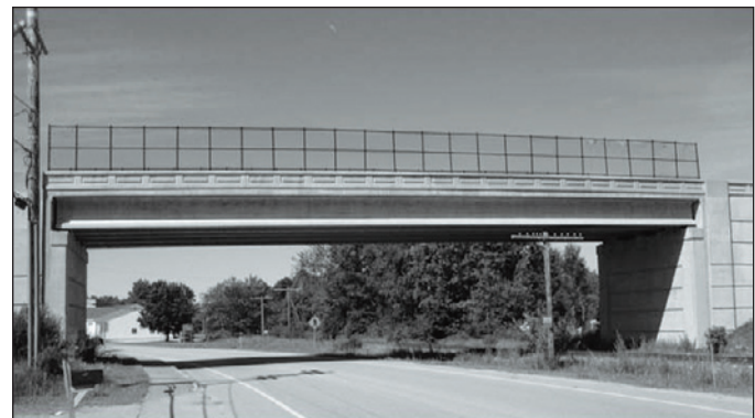
Figure 3-30: New Rollins Road Bridge, opened in 2000
