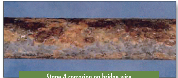
Stage 4 corrosion on bridge wire
