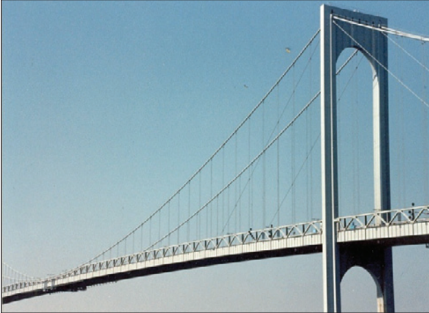
Figure 3-7: Whitestone Bridge in the 1980s
