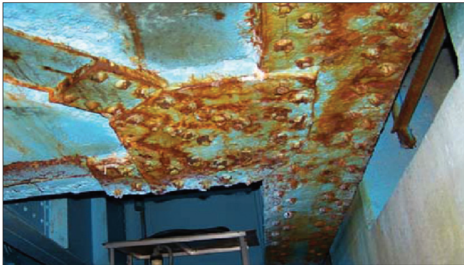
Figure 3-3: Corrosion of a steel member.
