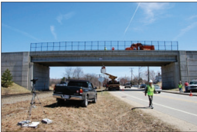
Figure 3-32: Digital Camera Set up for Digital Image Correlation at Rollins Road Bridge
