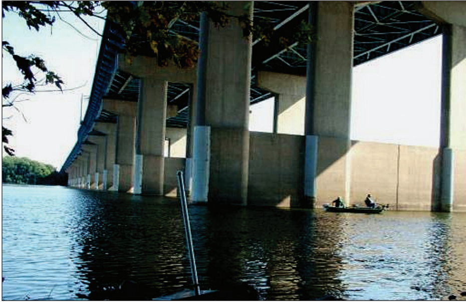
Figure 5-25: Bridge located near Harrisburg; southbound span shown here.
