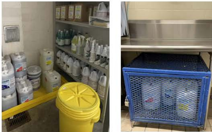
Exhibit 1. Chemical storage areas for SLIPC's Food Service Department. Chemicals are in original manufacturer's containers, labeled with contents, and stored correctly (left); chemicals are in locked storage cabinet (right), as observed by OIDO on October 26, 2022.
