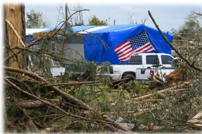
Figure 31: Tornado Damage in Mississippi
