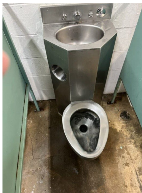
Exhibit 6. Discolored toilet in C Dorm with black and white spots inside (left) and black debris on privacy walls between the toilets in Unit 5 (right), as observed by OIDO on September 27, 2023.
