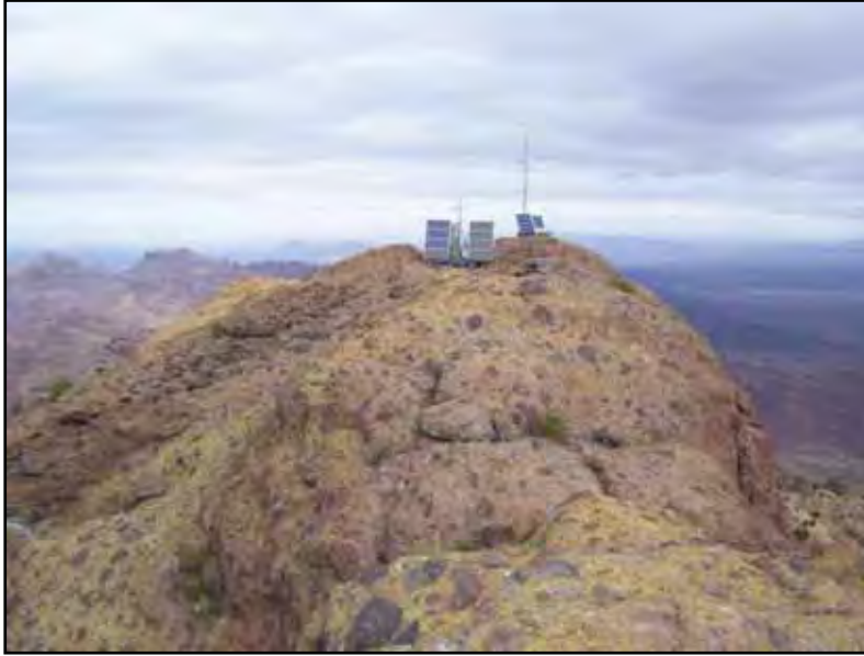
Photograph 5.13 Overview of TCA-AJO-091 looking east-southeast.
