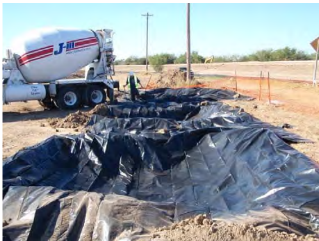
Concrete wash out pit, Hidalgo, TX
