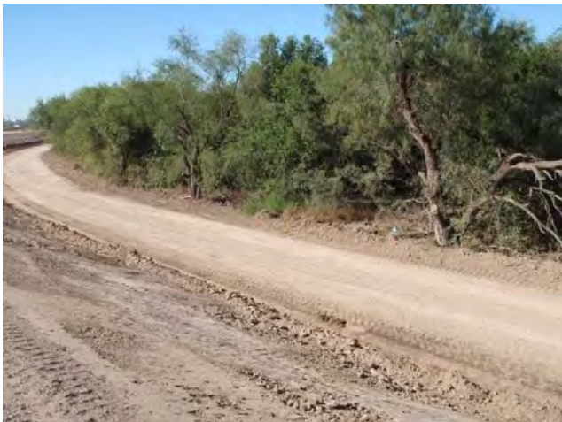
Construction corridor bounded by berm, Hidalgo, TX
