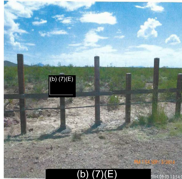
Vehicle Fence – Post/Rail
