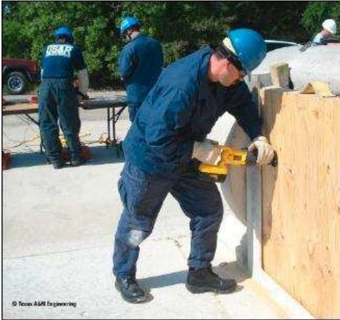
Figure 3. A SME performs a breach cut on a simulated wall panel.
