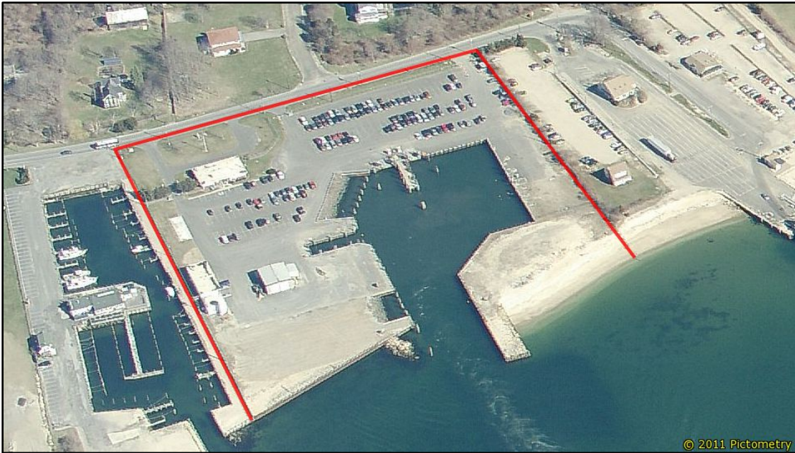
Figure 9. Aerial View of the Orient Point Facility
