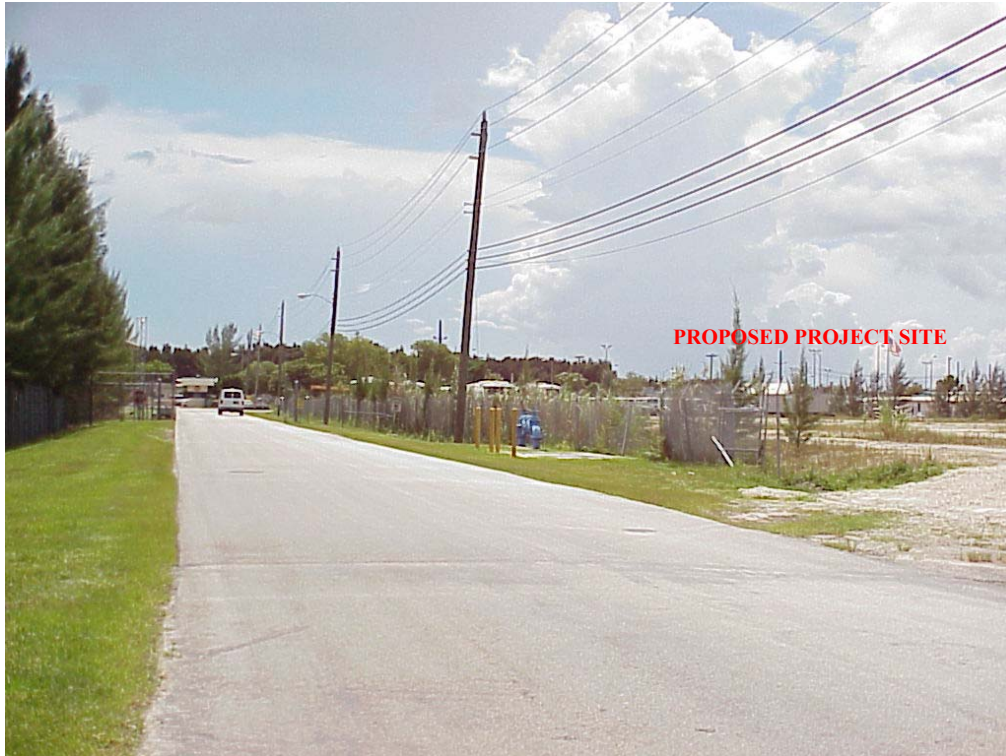
Exhibit-3 The Krome SPC service road and proposed development area on the right
