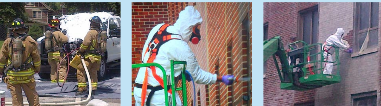
Columbus first responders demonstrating decontamination techniques using foam during the Wide-Area Urban Radiological Containment Mitigation and Clean-up Toolbox Technologies demonstration.
