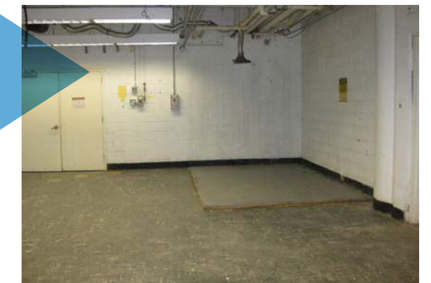
Radon Chamber after.
