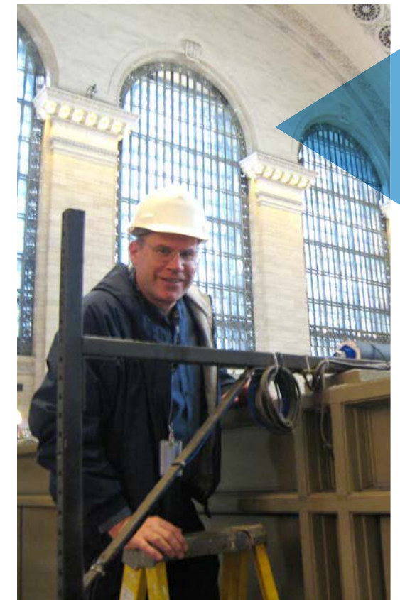
Engineer Brian Albert installing REMS sensors at Grand Central Terminal.
