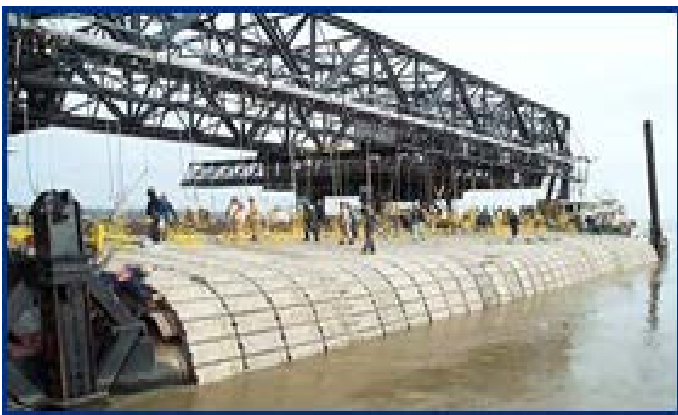
Protective mats being installed in 2010.
