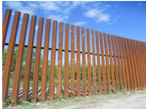
Photograph 3-2. Primary Pedestrian Fence Design in Cameron County
