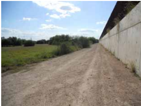
Photograph 3-1. Concrete Flood Protection Structure/Concrete Fence Design in Hidalgo County
