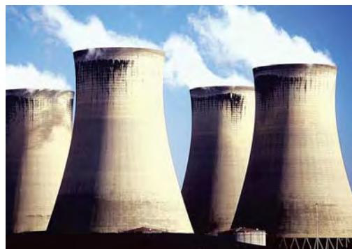
Nuclear Power Plant Cooling Towers
