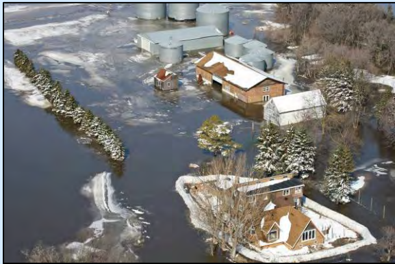
Halstad, Minnesota, March 29, 2009: Flooded farms and rural communities in Norman County, Minnesota, adjacent to the Red River of the North were affected by this year's record flooding in March, 2009. It was declared a major disaster on March 24, 2009.
