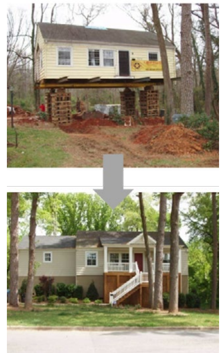
[Figure 24] Example of structure elevation
